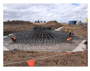
After the new reinforcing was in place (pictured), the new foundation was poured on the 11th of February and needed nearly seventy concrete trucks coming from Geelong and Colac to deliver the nearly five hundred cubic metres of concrete needed for the foundation.
